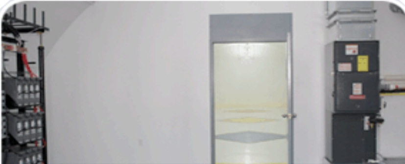
BUNKER MECHANICAL ROOM
