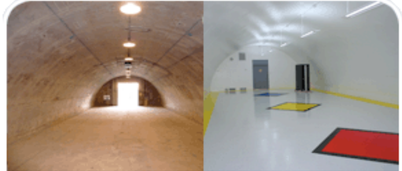
BUNKER INTERIOR - BEFORE AND AFTER
