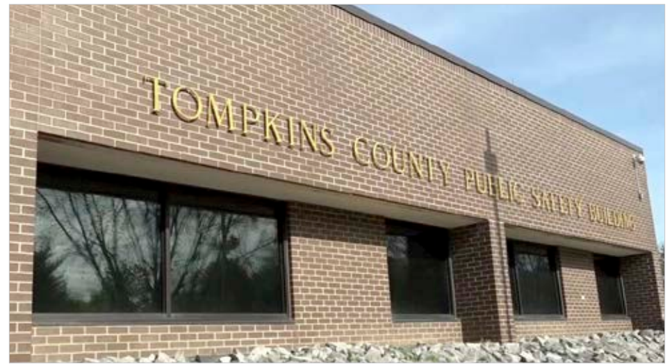
The Tompkins County Legislature is forming a task force to consider making renovations to the public safety building, which houses the county jail. (Photo Credit: Tompkins County)
