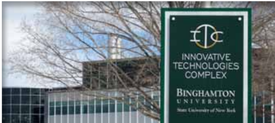
The initial building in Binghamton's Innovative Technologies Complex
