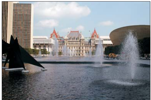
The Nelson A. Rockefeller Empire State Plaza. Photo courtesy of NYSOGS Michael Joyce.
