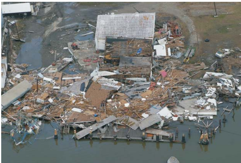
Cameron Parish, LA, after Hurricane Rita
