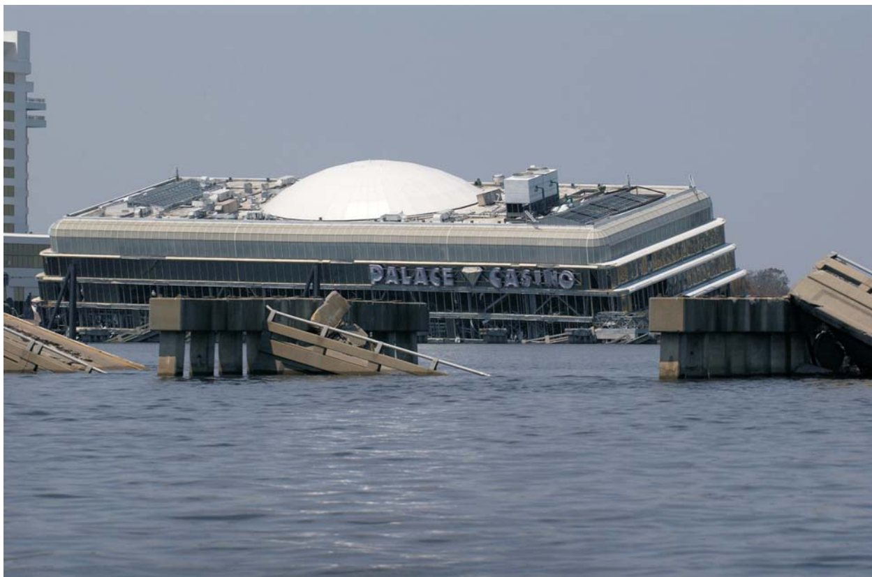
The Palace Casino in Biloxi, Mississippi, is partially submerged and severely damaged.
